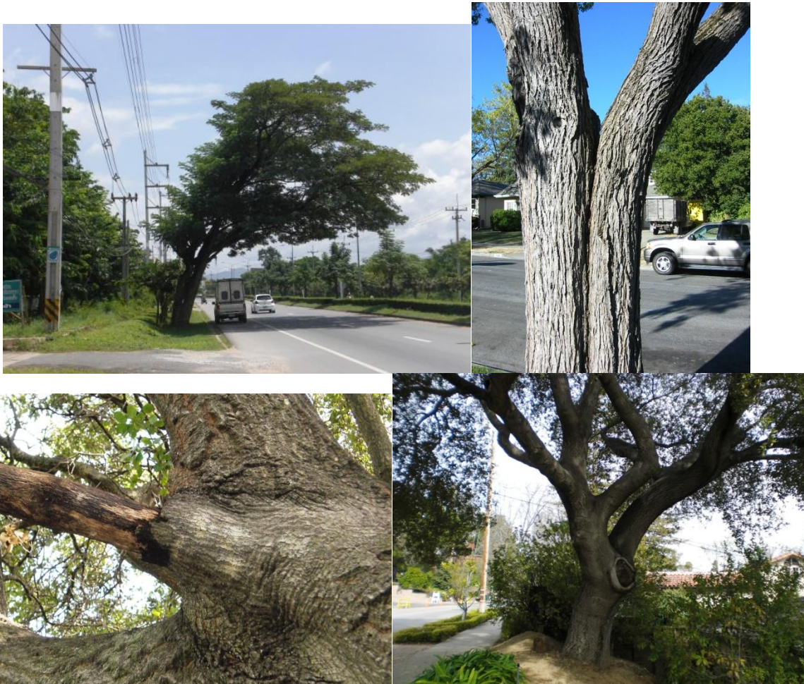
Some structural defects (clockwise from top left): 1. Imbalanced weight distribution, leaning. 2. Co-dominant stems splitting apart. 3. Large deadwood. 4. Large wound at critical location.
